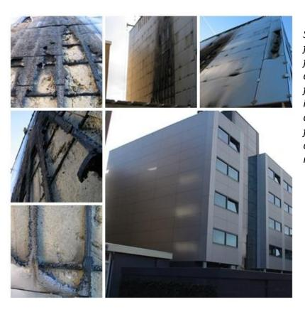
Some pictures of a cladding fire in 2006. As a result of a fault of a roofer, a hpl cladding on a wooden frame, which was completed in 2004, went on fire. The cladding partially went up in flames. The bonded fixture on the wooden battens maintained.
