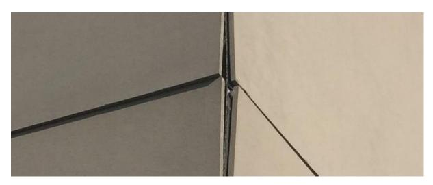
The stresses that occur are reflected in the "curling of the ears" of the façade panel. As a consequence, there is a permanent tensile stress on the glue joint, eventually resulting in an adhesive fracture and / or delamination of the glued substrates located at the corner(s) of the façade panel.
